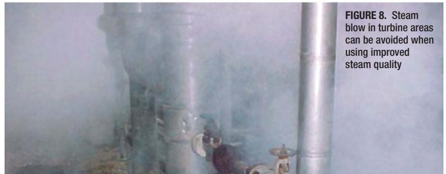
**FIGURE 8.** Steam blow in turbine areas can be avoided when using improved steam quality
